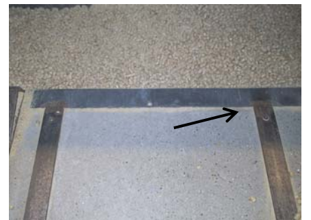
Rails welded together with flange of scrape system.
