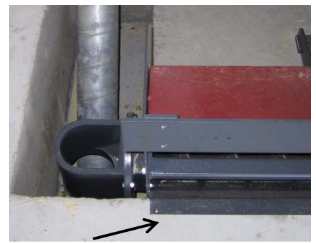
The flange is placed on the edge of the pit
